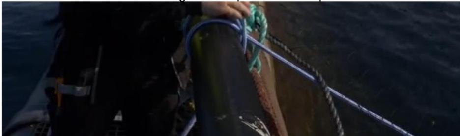
5. The pulley below the top ring must be tightened as much as possible such that it has no slack to move. This will prevent it wearing through the rope too quickly. **This must be included as a checklist item when inspecting pens.**
