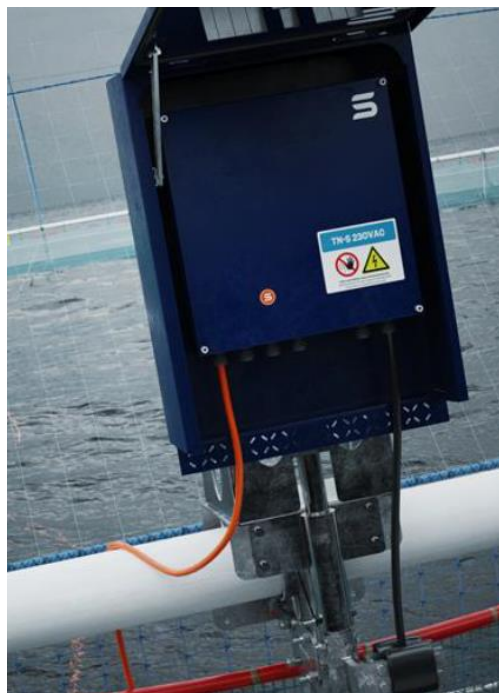
Figure 2: The control cabinet is supplied with a protective cabinet.
